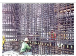
Fig. 8. BauCages® Installed with BauSplicegrids<sup>TM</sup>
