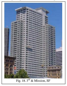
Reinforcement System proved to be the answer to the need to hold very exact dimensional tolerances so that the precast elements could be fit together rapidly and the prestress strand and mild reinforcement easily installed.
